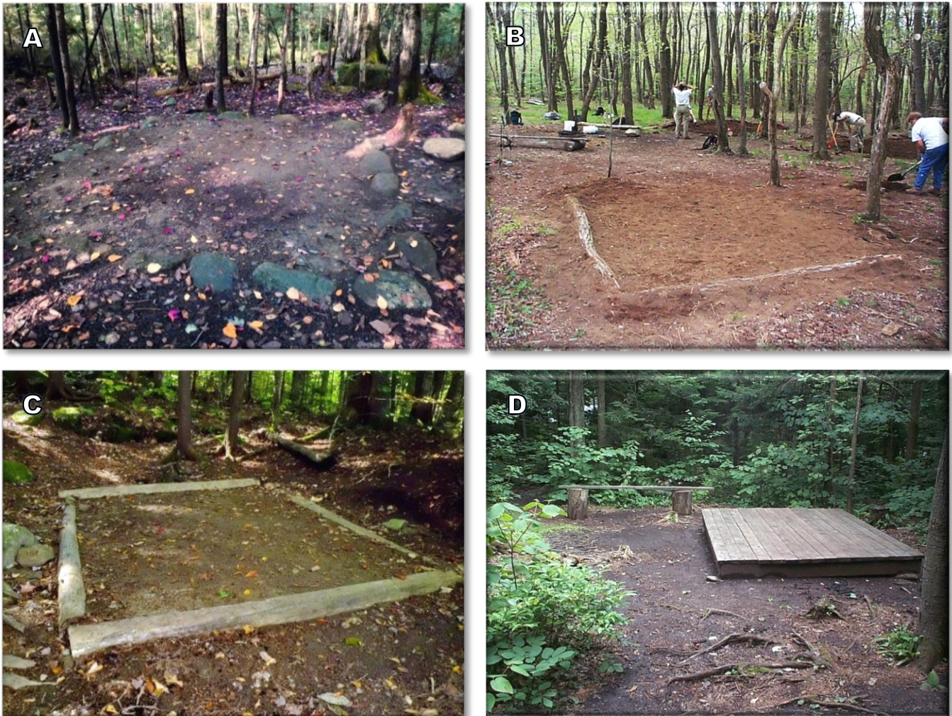
Figure 13. A) Rock-lined tent pad, B) Embedded logs pinned with rebar, C) Wood-lined tent pad, and D) Wood-decked tent platform.
